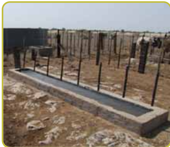
Photo 66: Up to 1500 cattle can drink from a 5m-long trough if the trough re-fills quickly
